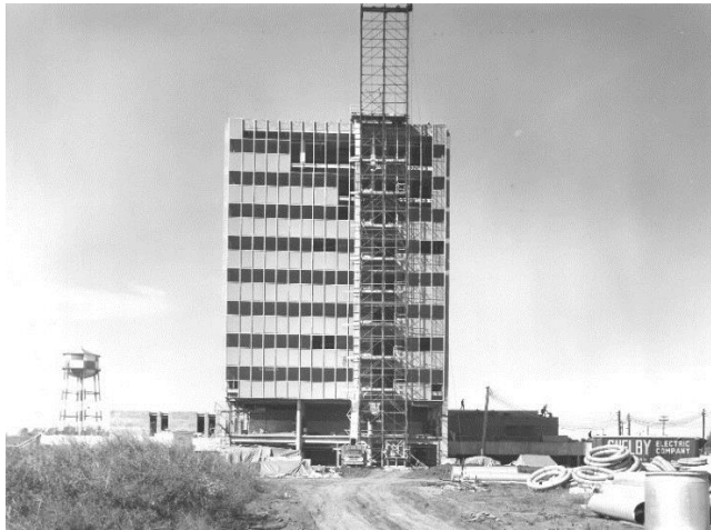
Construction of 4200 (Photo & Article courtesy The Marshall Star)
